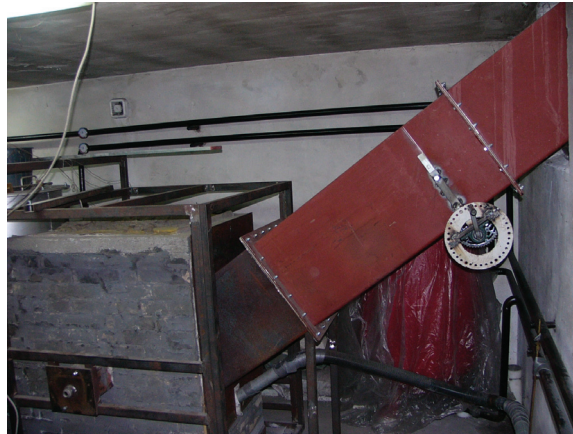
Fig. 4. Inclined fuel feeding
