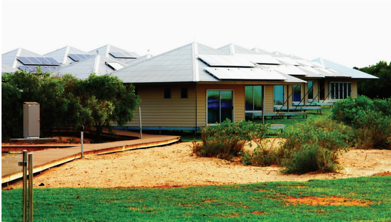
Fig. 18. Eco resort villas with photovoltaic panel installation
