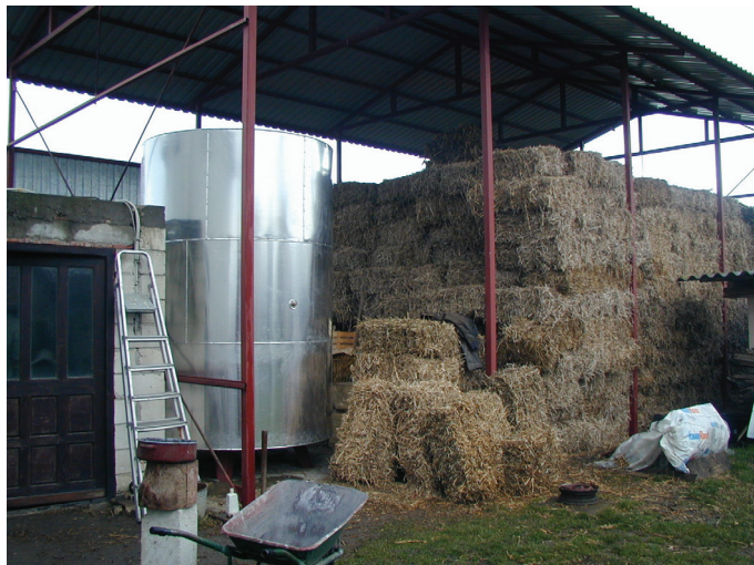
Fig. 6. Heat accumulator (thermal reservoir)
