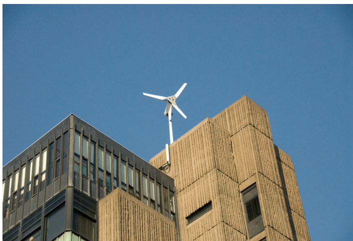
Fig. 6. Roof mounted turbine
